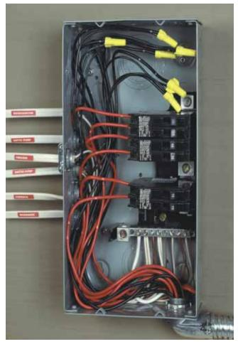
Note: A 6-circuit, 125 amp panel was used for illustration purposes only. EmerGen Switch® Owner's Manual
